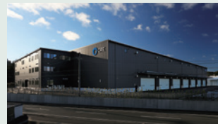
Example:LogiSquare Kakegawa (Shizuoka Prefecture)
