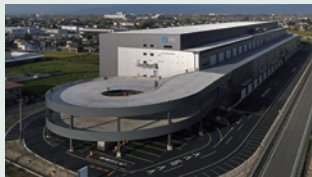
Example:LogiSquare Ichinomiya (Aichi Prefecture)
