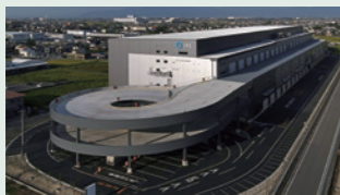
Example:LogiSquare Ichinomiya (Aichi Prefecture)
