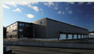
Example:LogiSquare Kakegawa (Shizuoka Prefecture)
